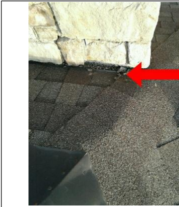
A small piece of brick maybe missing on the corner of the chimney.
