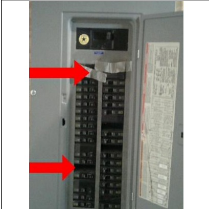
There are several missing Breakers in the Box. The Open Spaces should be filled in with blanks. The taped off Breakers at the top of the box we're for hot tubs which are no longer in the building.
