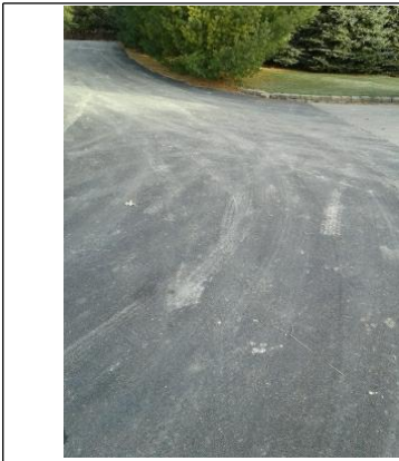
The blacktop driveway is in satisfactory condition.
